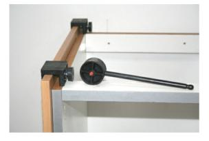
This picture show the trim line. Anything below this line is waist. Tip **never** cut out Your line as this is a reference. Plain or cut to the centre of the line. Seal exposed edges and fix Panel in position. Attach clamps as shown and make sure that you have no daylight between the Clamp top and the end panel top
